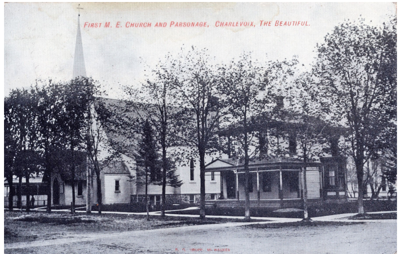
Right: The Methodist parsonage on the Clinton Street corner, built 1880. It survived well past the middle of the 20th century.
