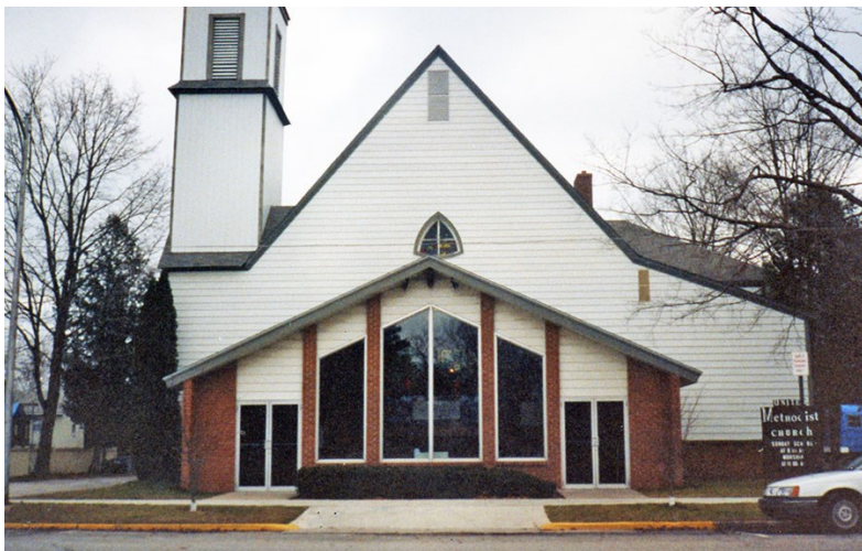
Left: This remodeled entry appeared in 1972. The lengthy, 10,000 sq. ft. fellowship hall addition, with kitchen, restrooms, and five classrooms, would appear to its right, on the parsonage land, in early 1997. Another pointed steeple, still there, also made its appearance around the same time as part of a massive, year's long renovation and restoration job.
