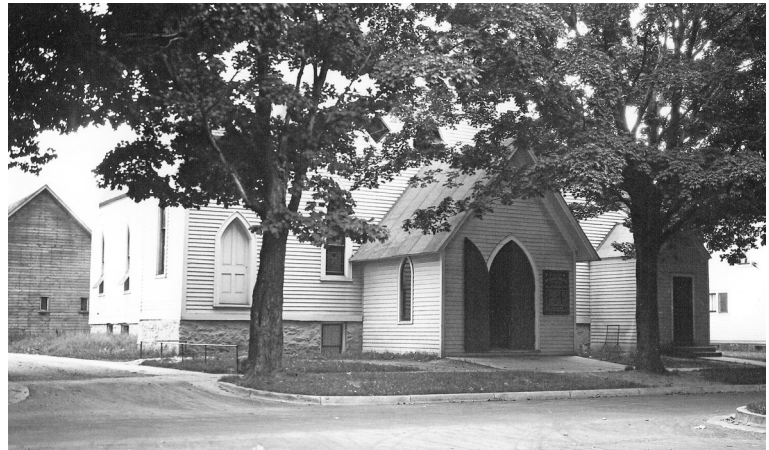
Above: Close-up of the original Gothic-arched entry, with the church's barn appearing behind it on the alley.
