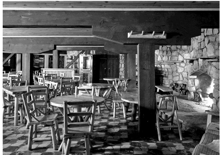
On the lower lounge level, Earl retained the mill's original pillars and their transverse extensions under the main floor. Still today, these extensions (where the coat/hat rack is positioned above) are low enough to cause serious head thumps to those not paying attention.
