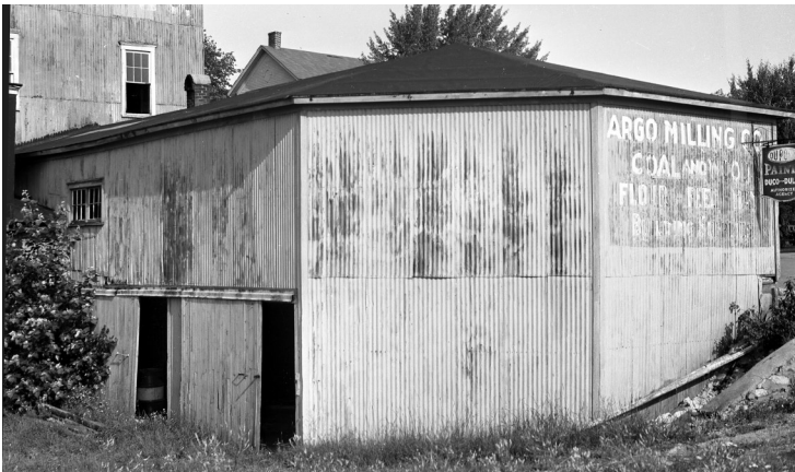
The main shed beside the highway, made of corrugated iron sheeting
