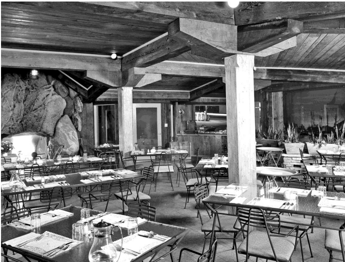
Two of the original foot-square maple pillars from the old mill that Earl re-incorporated into the new structure as either supports or embellishments, each with its own unique notchings and cut marks, here in the main dining room
