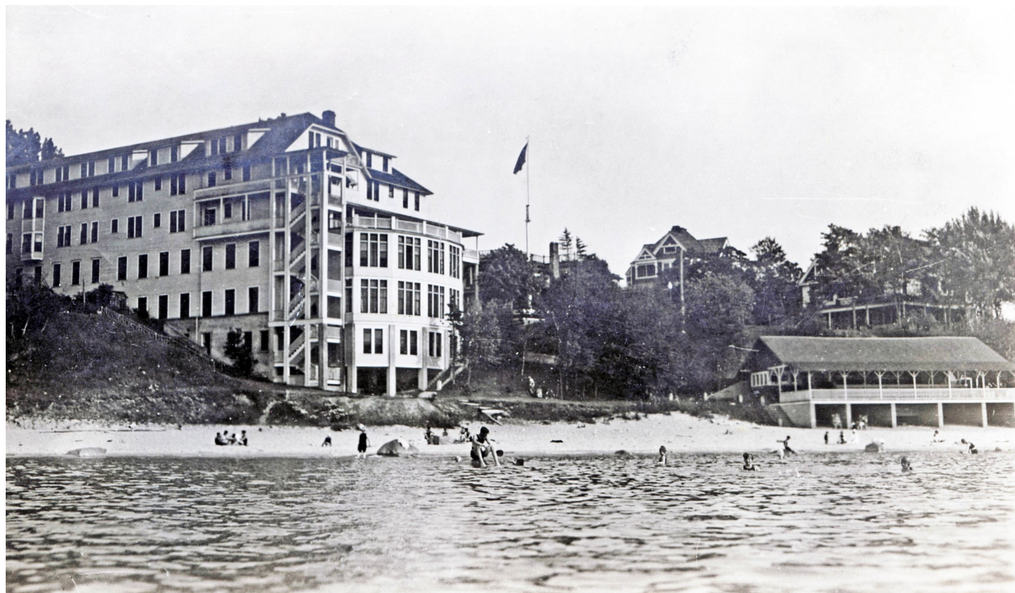
Seven stories, the tallest building ever constructed in Charlevoix. Beachside social pavilion at right
