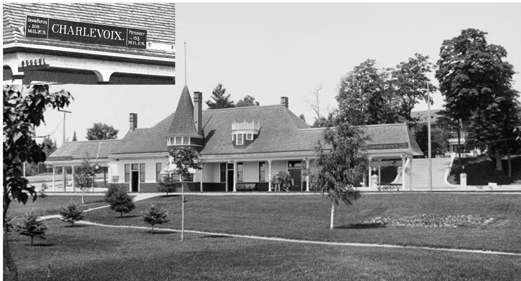
Landscaping flourishes, post-1898. Wide staircase up to 250-room The Inn hotel is seen at right. Sign on corner eaves: Grand Rapids, 209 miles; Petoskey, 15.5 miles
