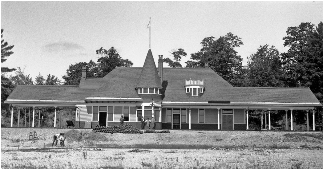
Just prior to completion, with drainage pipes stacked beside the tracks
