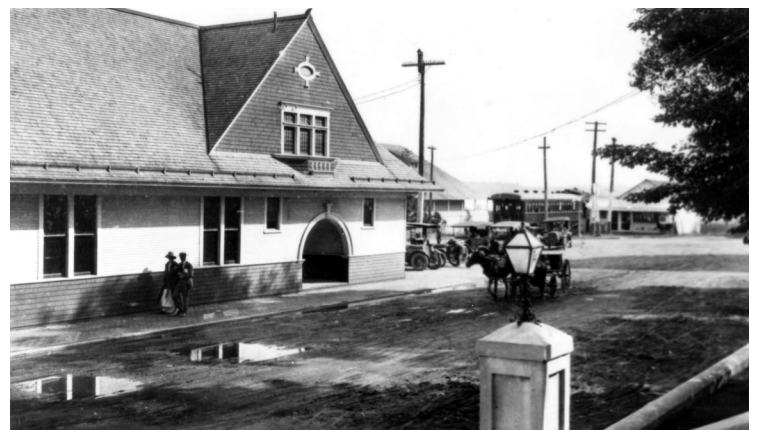
The main entrance to the depot consisted of an archway open to a recessed vestibule that held two doors to the interior on the inside. After too many winters of snow piling into the west-facing gap, a single outside door flanked by two stained glass windows was installed to enclose the archway and block the vestibule from the elements.
