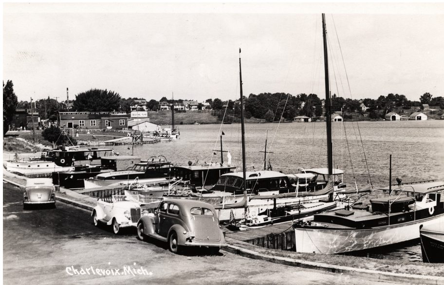
Paved access road with cement curbing, late 1930s
