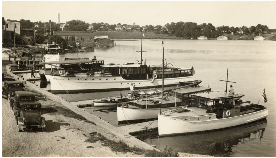
Charlevoix's first five pleasure boat slips, mid-1920s, with dirt access road for cars
