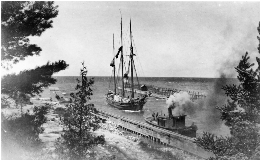
A tug brings a schooner, with sails furled, into safe harbor, ca. 1900. Note the wooden catwalk on the north pier, a popular pedestrian promenade structure, in place 1885-1904 when it was replaced by a metal catwalk.
