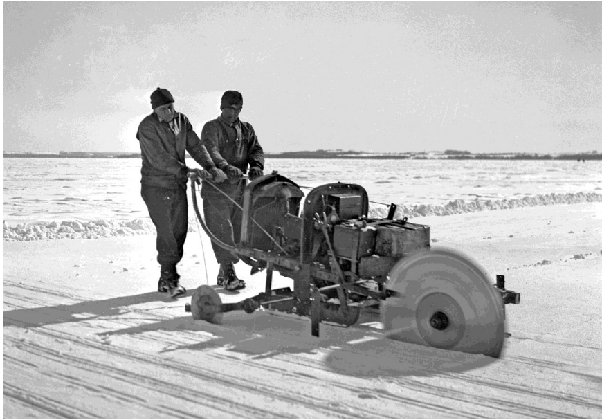
Ice cutting on Lake Charlevoix with a converted automobile engine.
