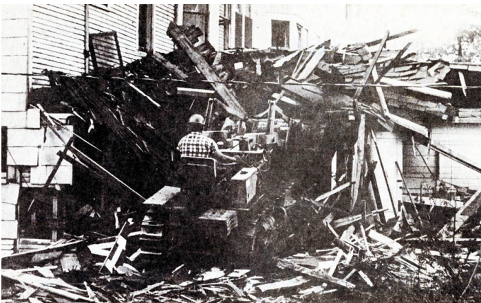
Bulldozers apply the major touches
