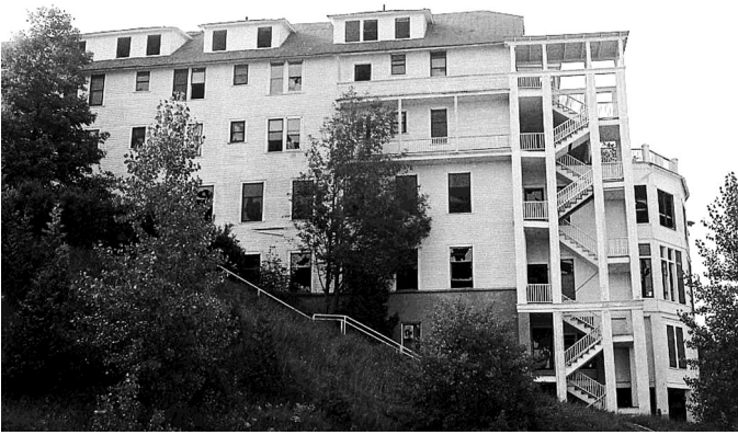
Vacated Beach Hotel, with one staircase gone, broken and missing windows that allowed in the elements
