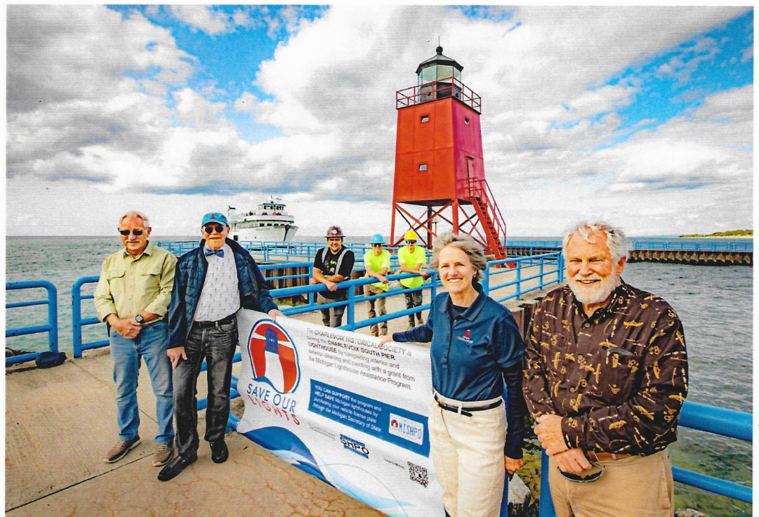
The South Pier Lighthouse project to repair and paint areas of the interior and exterior got underway on September 8, 2025, and is expected to continue into October. Blas Tek LLC of Shelbyville, MI, was awarded the contract. Pictured with the Lighthouse Committee are Blas Tek employees. (l to r): Mayor Lyle Gennett, Councilman Richard Spring, Ian Fillmore, Geno Wierckz, Zach Carlson, Denise Fate, Tom Darnton.
